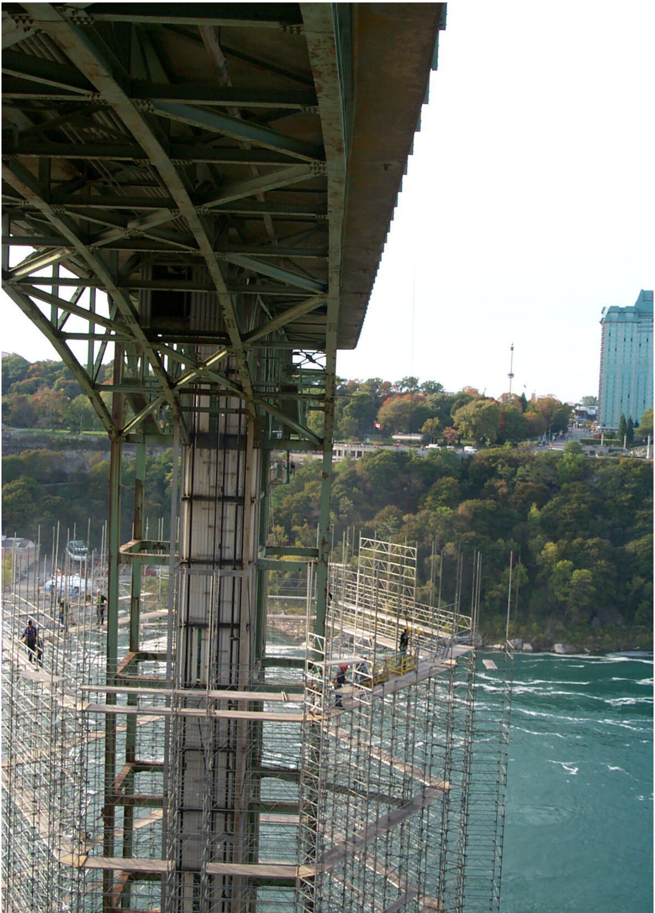
Scaffold Tower Installation
