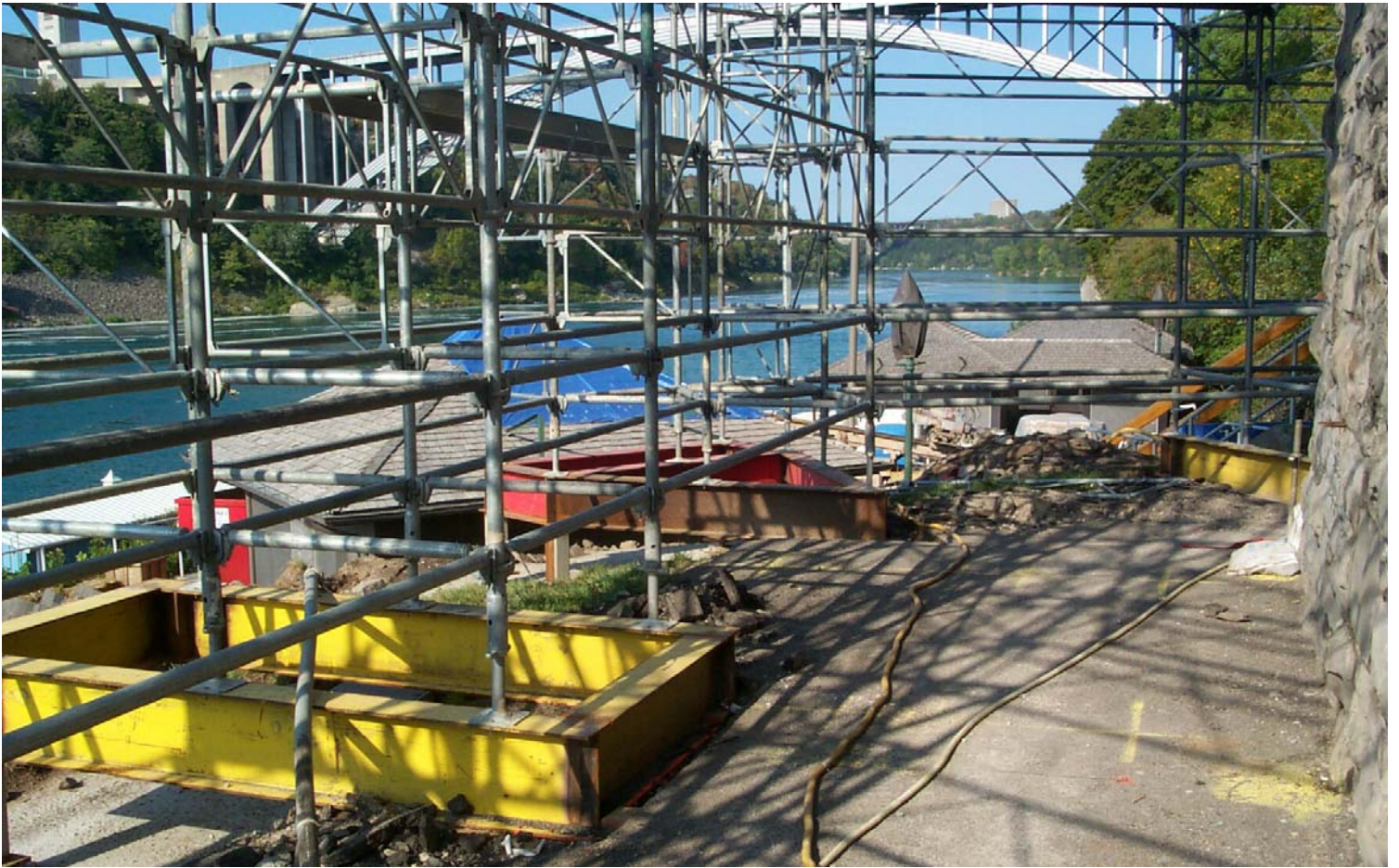
Structural Steel Tower Leg Base Supports
