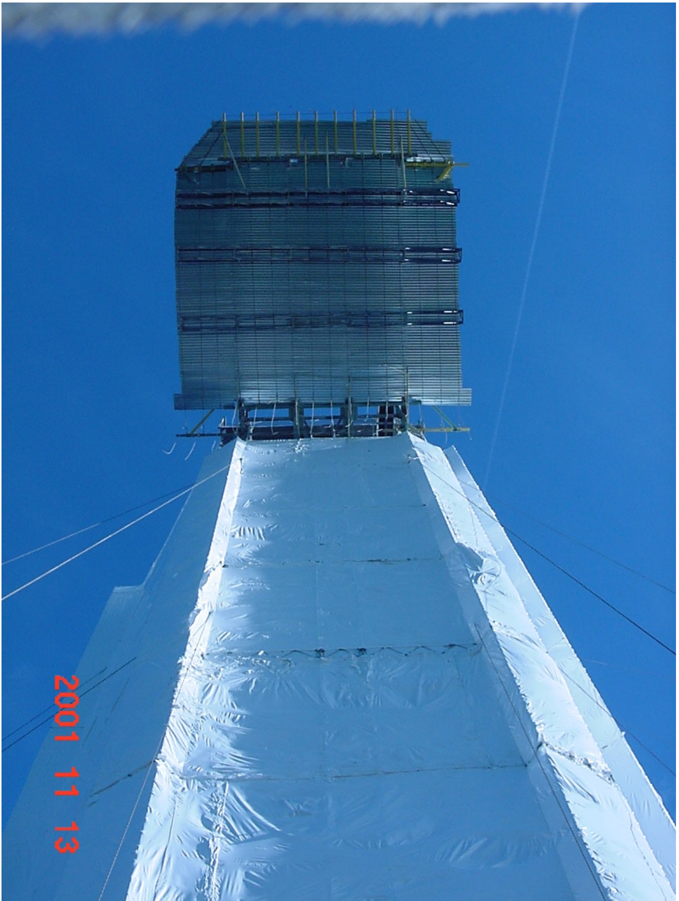
Scaffold Tower w/ Containment & Cable Supported/Metal Deck Platform
