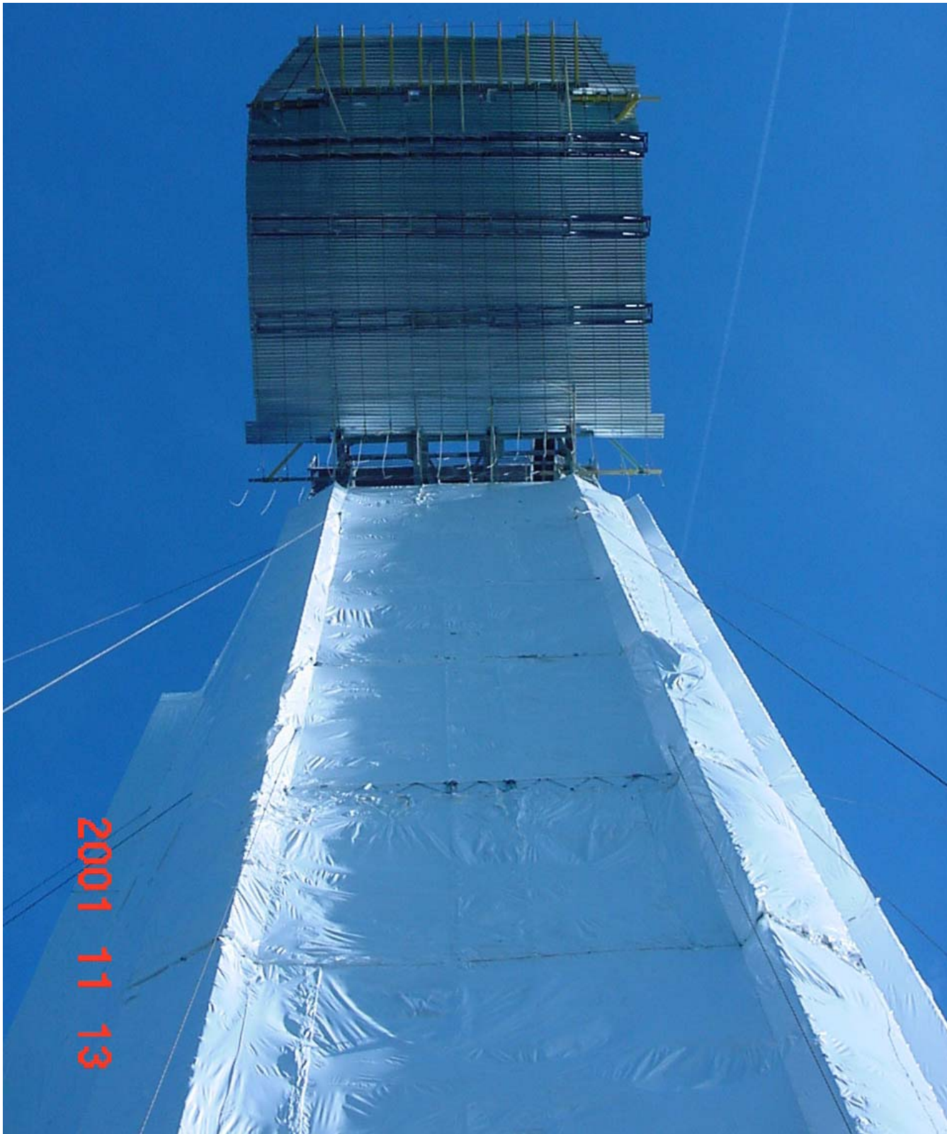
Scaffold Tower w/ Containment & Cable Supported/Metal Deck Platform
