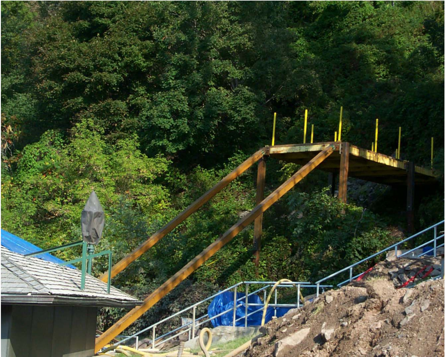
Telescoping Leg Drilling Platform For The Installation Of Rock Anchors In The Vertical Rock Face Of The Niagara River Gorge
