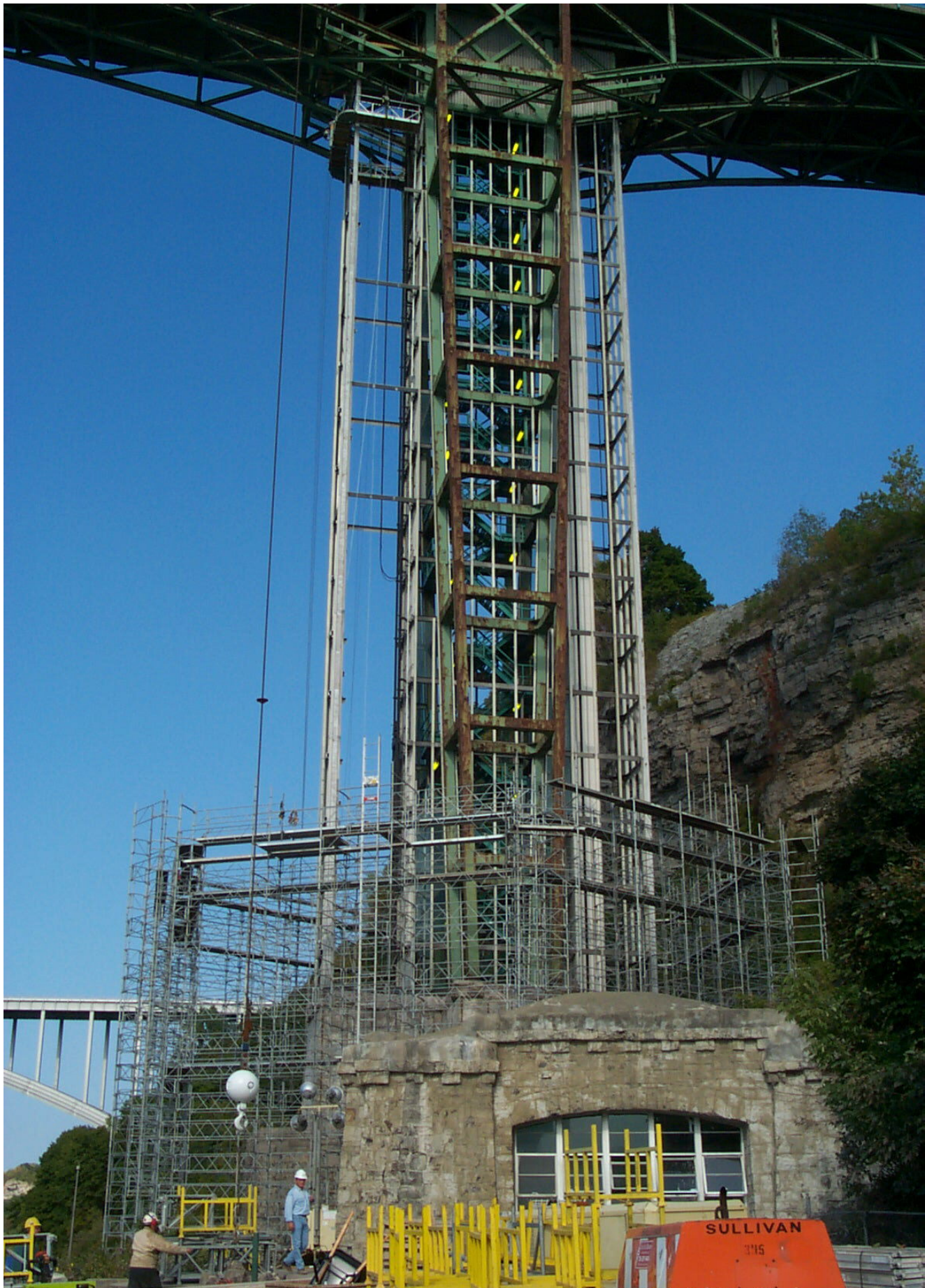
Beginning Of Scaffold Tower Installation
