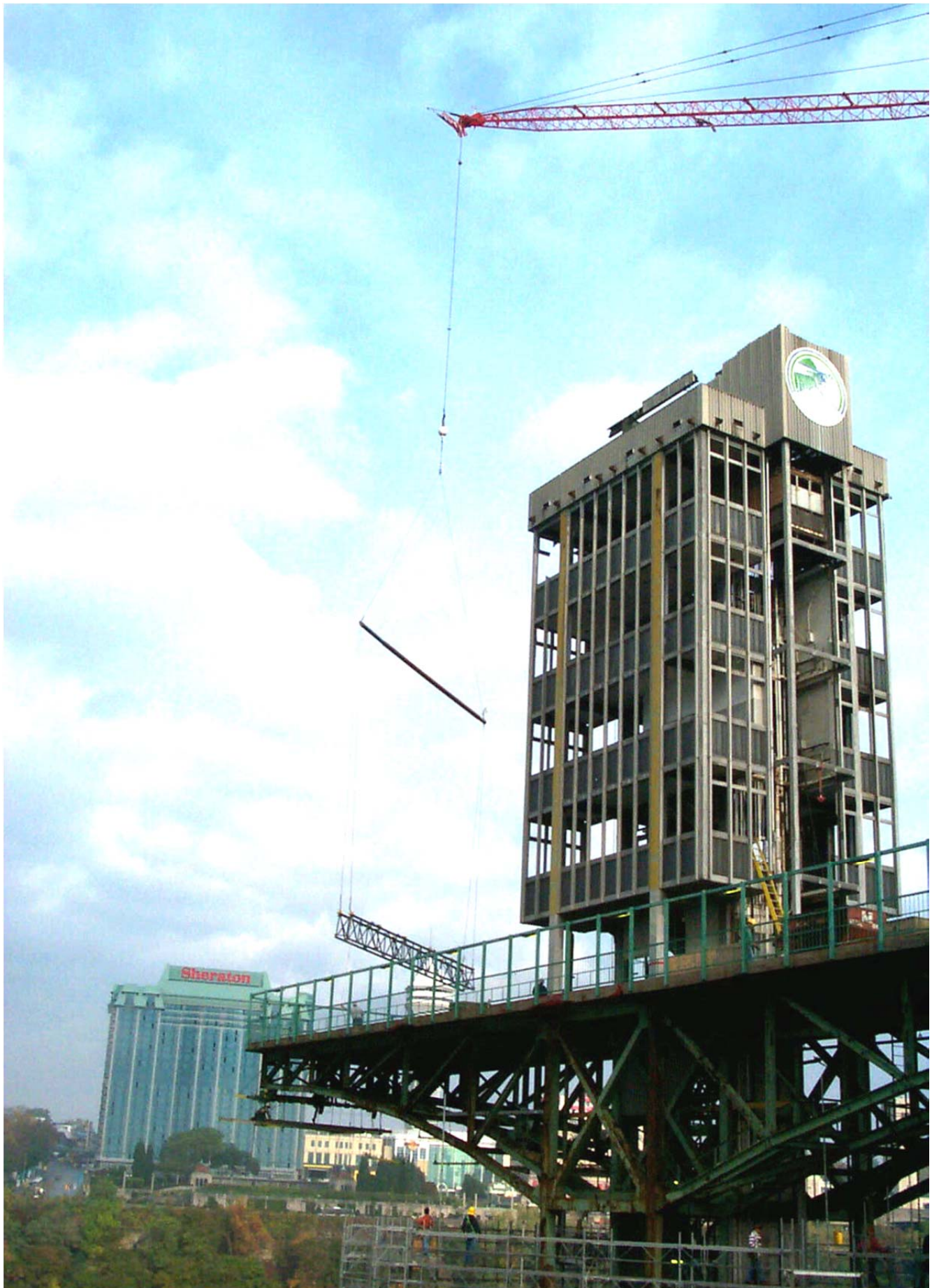
Main Cable Truss Support Assemblies Being Positioned In Place
