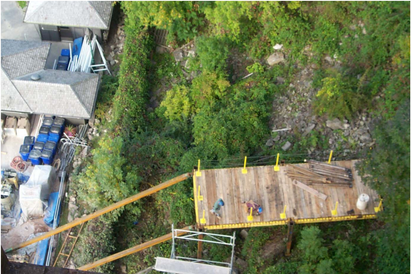
Telescoping Leg Drilling Platform For The Installation Of Rock Anchors In The Vertical Rock Face Of The Niagara River Gorge
