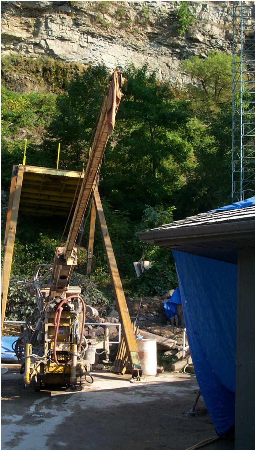
Drill Rig Ready For Placement On The Telescoping Leg Drilling Platform For The Installation Of Rock Anchors In The Vertical Rock Face Of The Niagara River Gorge
