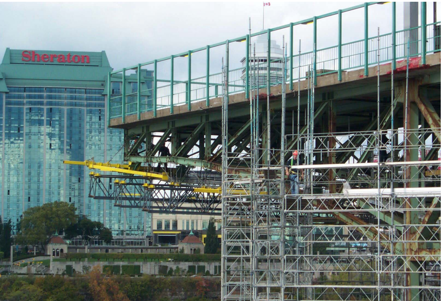
Main Cable Truss Support Assemblies In Place
