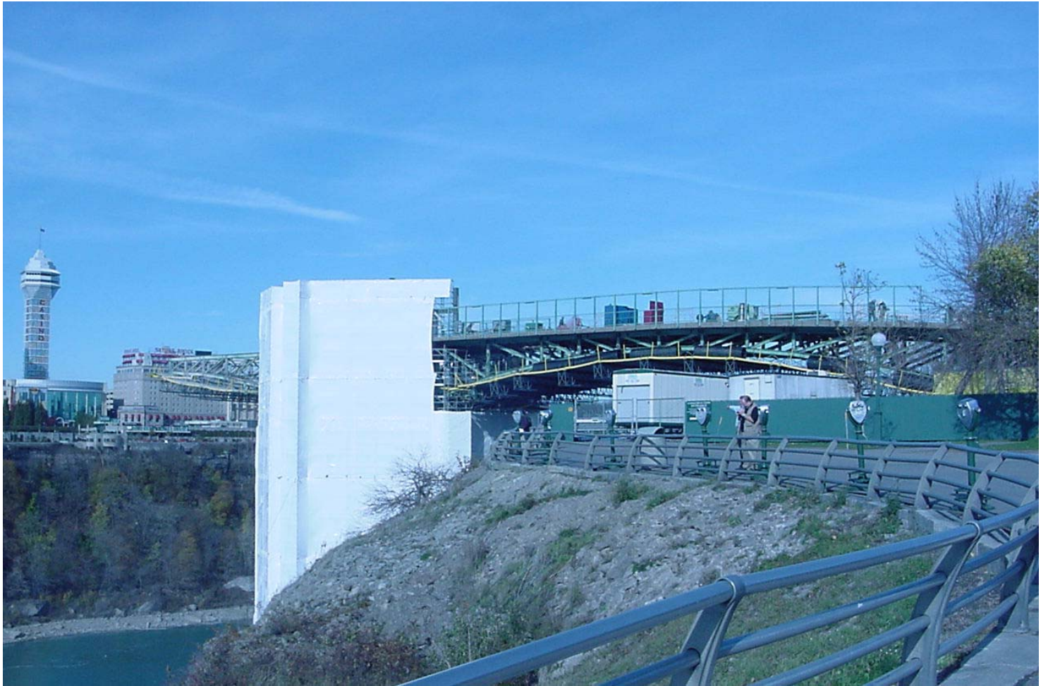
Scaffold Tower w/ Containment (Left) & Cable Supported/Metal Deck Platform (Right)
