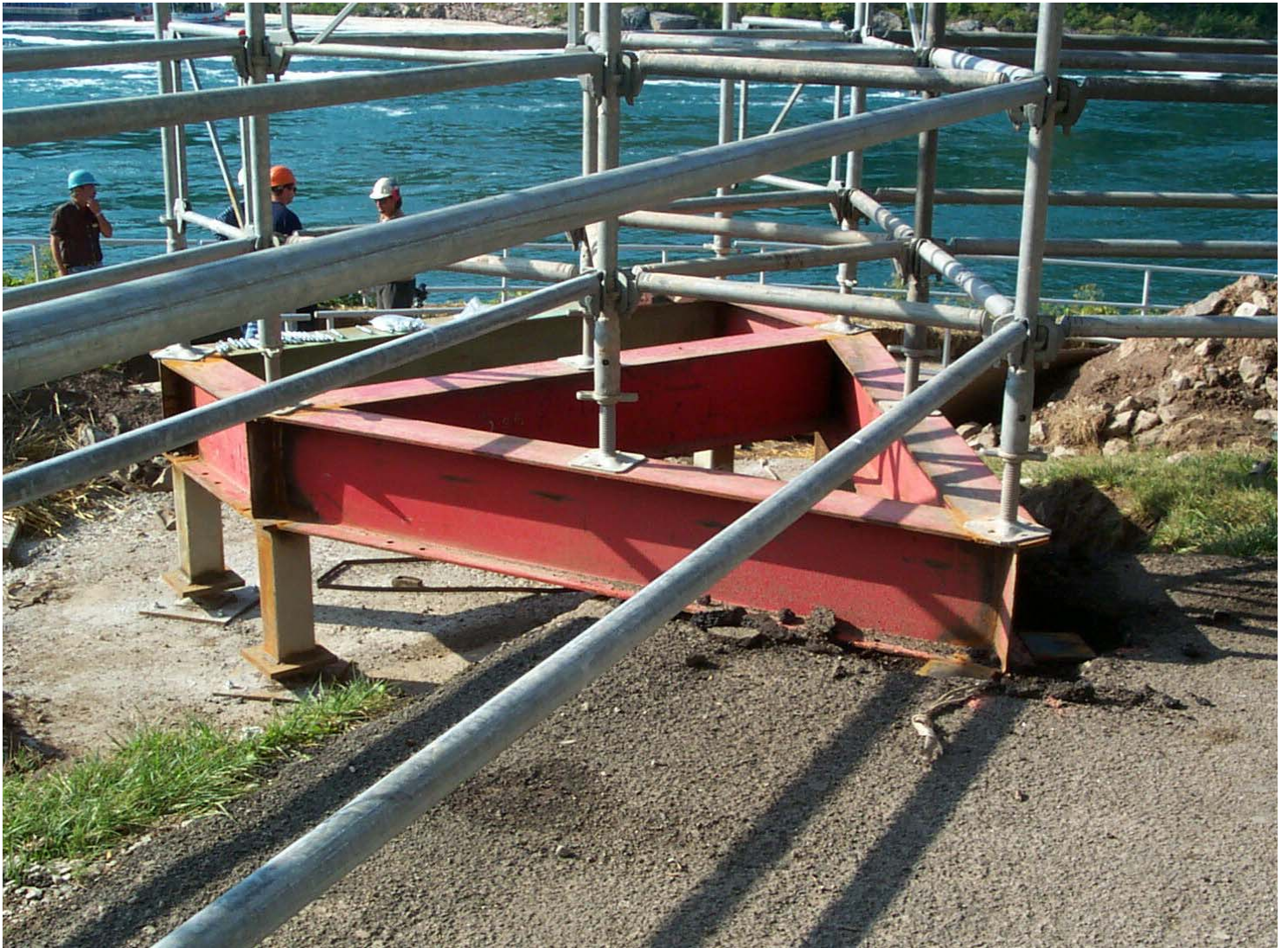
Structural Steel Tower Leg Base Corner Support
