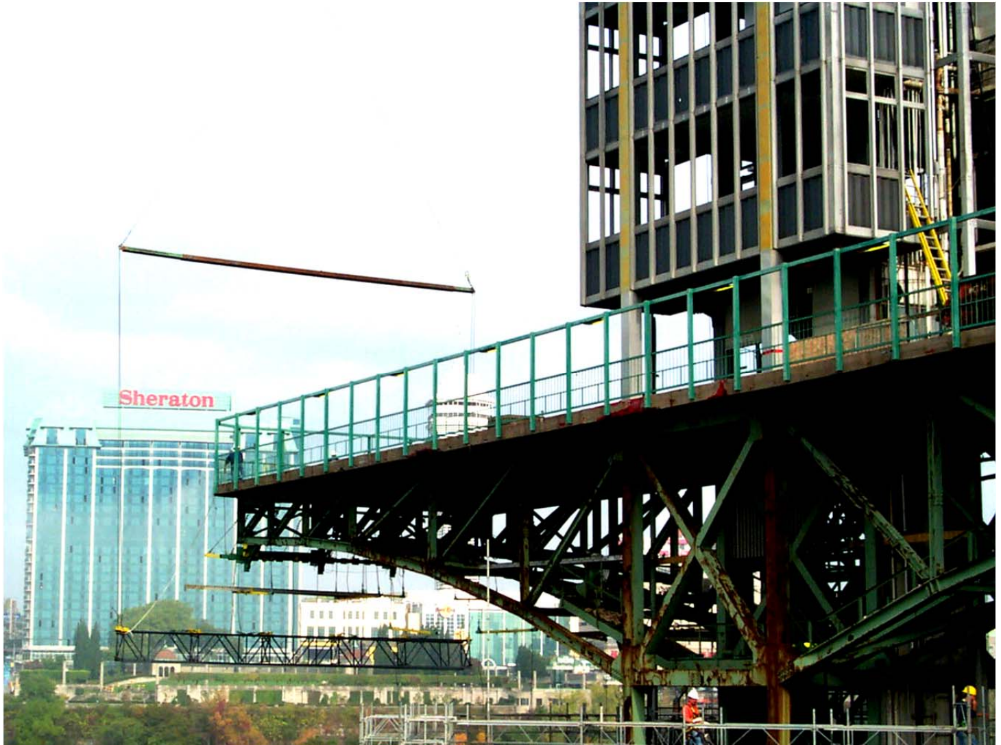
Main Cable Truss Support Assemblies Being Positioned In Place
